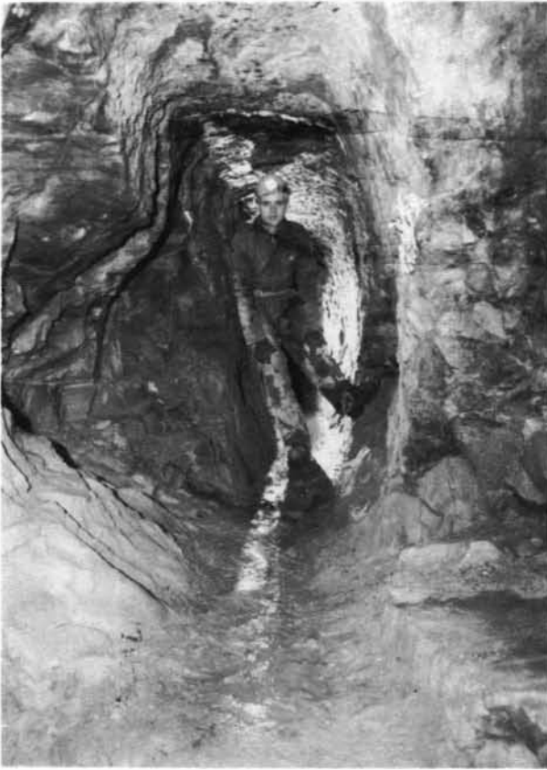
FIGURE 3. Pick-cut 'Roman' level crosscut above Lefel Fawr. Cwmystwyth, 1986. Photograph courtesy of Mr R.P. Jones, Welsh Industrial and Maritime Museum.
